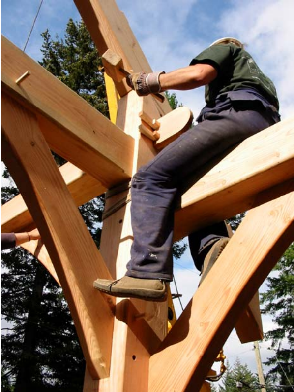
Finish Resurfacing / No Loosening
